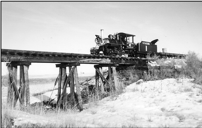
Engine No. 1, a 15-inch gauge "old time" 2-6-0, crosses trestle #2 on the Comanche Crossing & Eastern Railroad.
